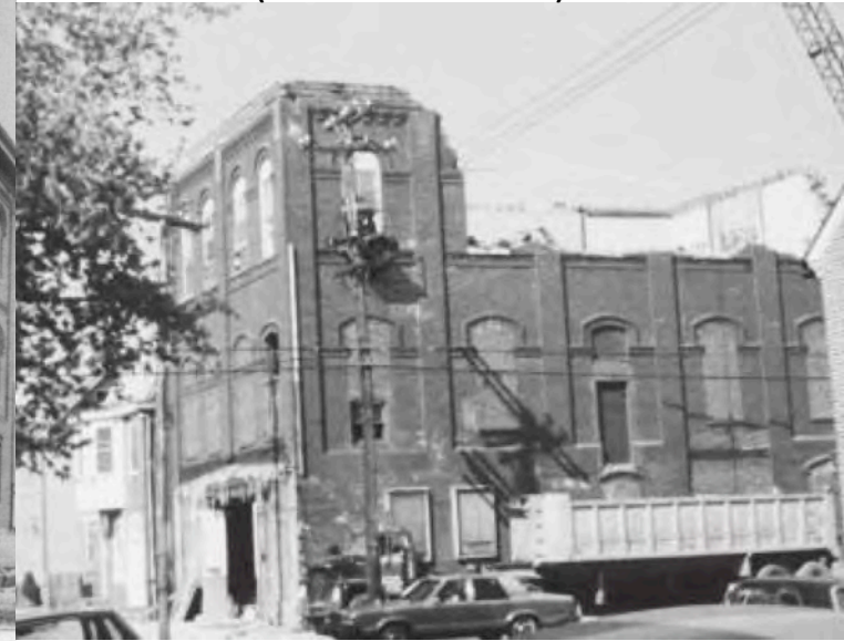
Demolishing the Earle Theater in 1983 (5 th & Delaware)
